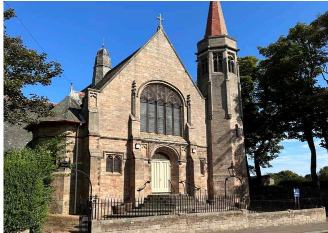
Crail Community Hall
